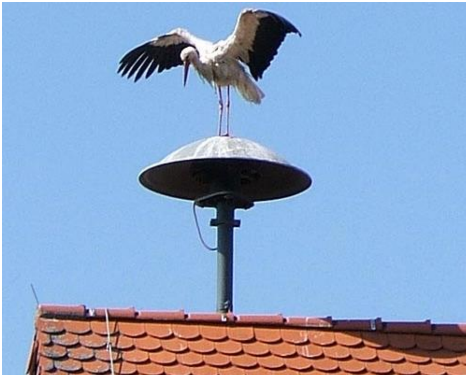
Figure 1: An electro-mechanical siren – Type E57 made by Hörmann in the 1950s
